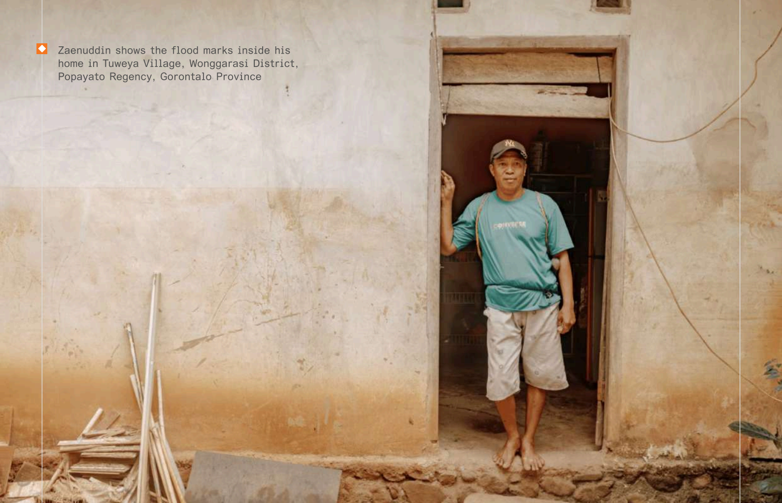
Photo 5. Aftermath of the June 2025 flood in Pohuwato Regency, Gorontalo, which affected around 1,235 people. Source: Trend Asia, 2025.
