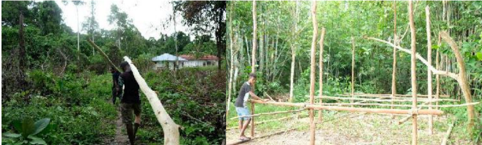
Figure 76 Working together to build a reading house
