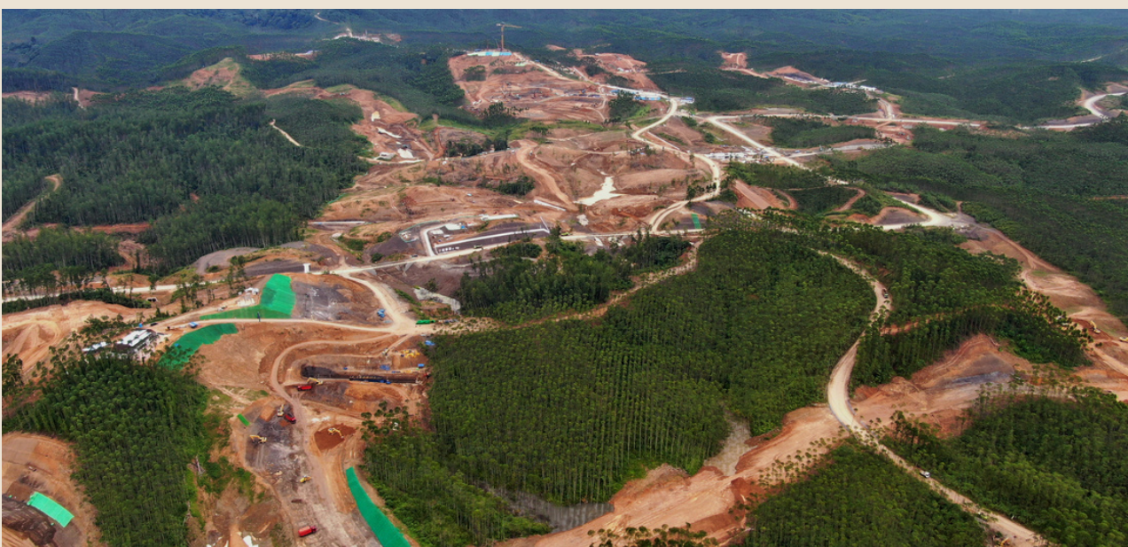
Aerial Pictures of the Construction of the Indonesian Capital Government Center (IKN)
